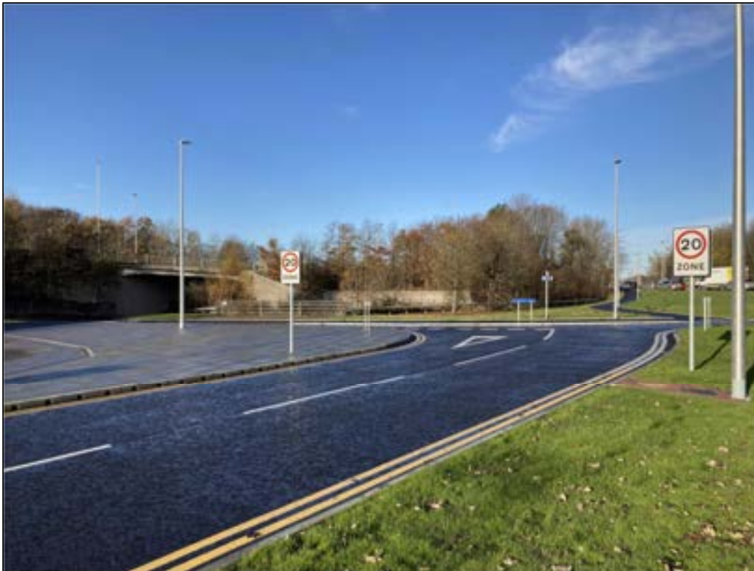
Figure 12 – New layout north of Old Meldrum Road (Site Walkover Photo)
