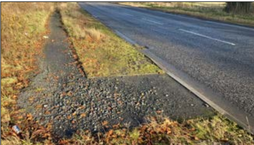
Figure 7 – Existing uncontrolled crossing
