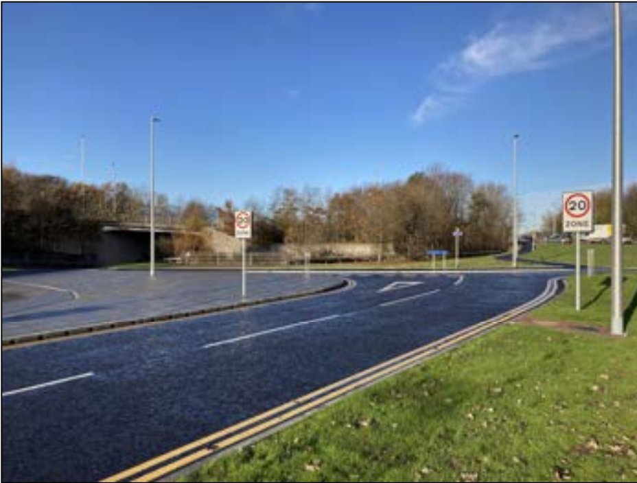
Figure 5 - New Layout North of Old Meldrum Road (Site Walkover Photo)
