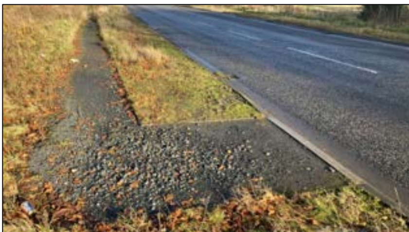
Figure 4 - Existing A947/B977 Connection Conditions (Site Walkover Photo)
