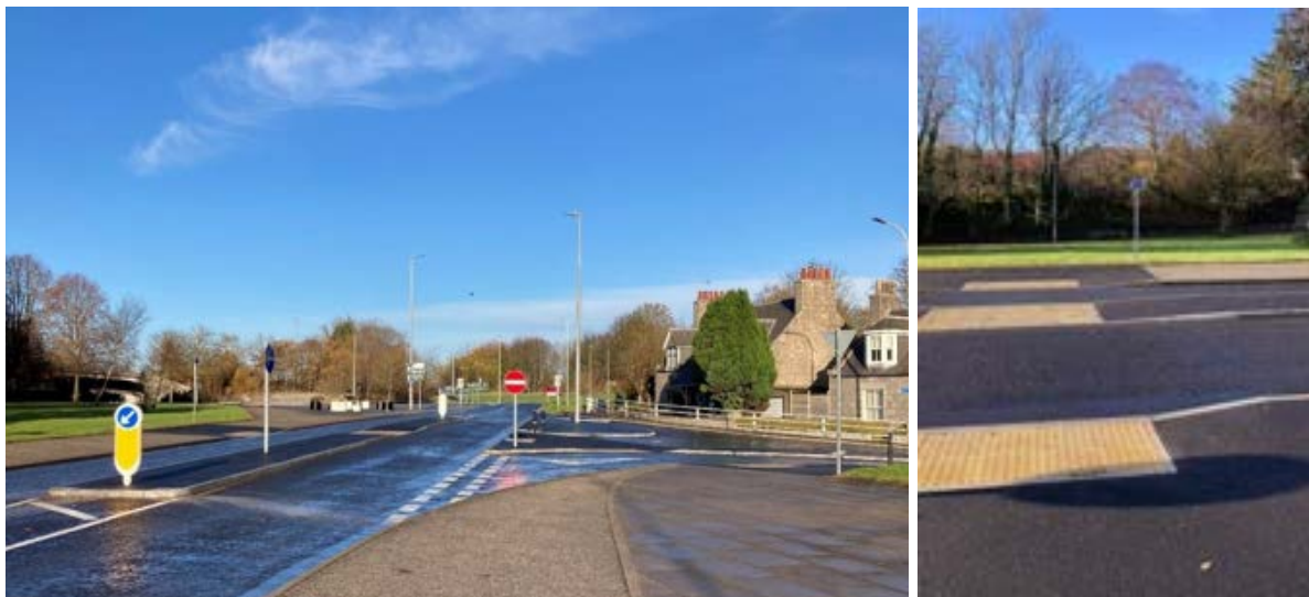
Figure 168 - New pedestrian crossing facility at the Old Meldrum Road/Mugiemoss Road Junction
