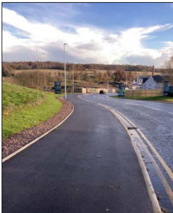
Figure 5 - Shared use footway adjacent to Mill Drive
