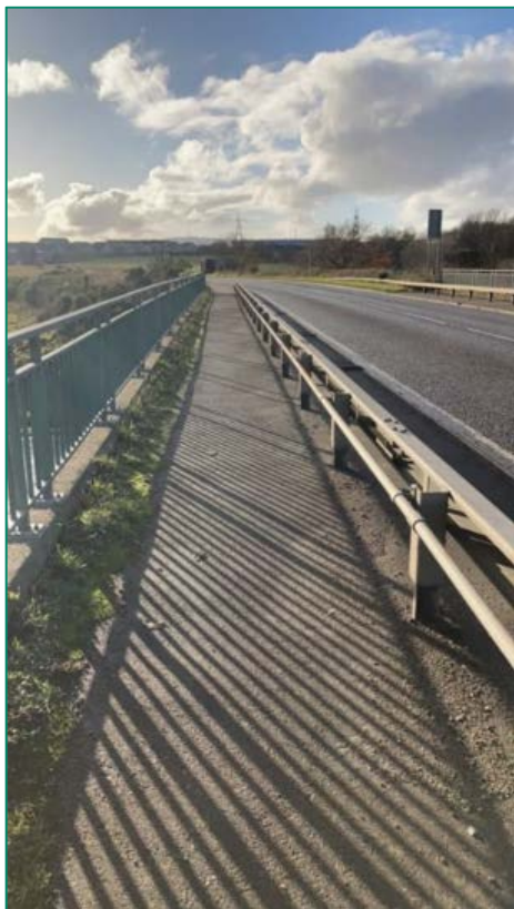
Figure 203 - Existing VRS set-back on Parkhill Bridge and diagram illustrating VRS set-back measurement (Source: DMRB CD 127)
